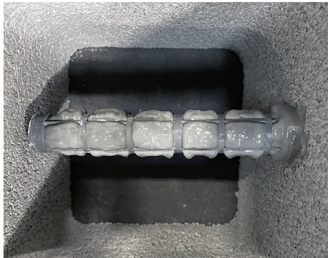
Specially sized holes in Opti-Mesh screens allow for adhesive to seep out at the appropriate location at the hollow portion of the CMU to create a better bond to the face shell.
